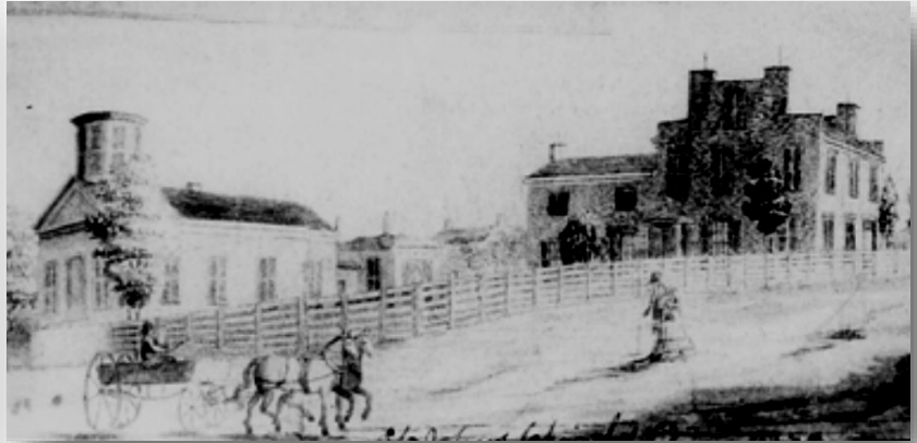
The original church building (built in 1838) and rectory (built in 1844).
